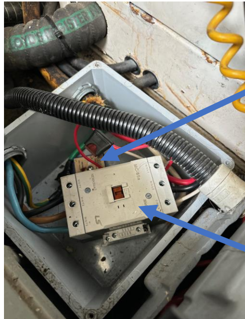
DIAGRAM C: Generator AC Relay box
